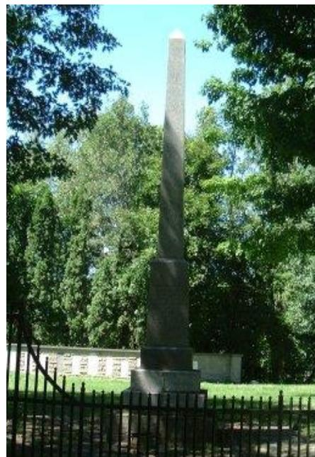
Due to its age, the monument is listing and needs to be levelled. The original limestone bases have badly cracked and need to be entirely replaced in order to prevent further damages to this important monument. In addition, the flagstone walkway, installed in 1956, shows signs of heaving due to frost and tree roots, and in many areas poses a tripping hazard to any visitors into the cemetery grounds. This again poses insurance risks to visitors so the entire walkway must be removed and levelled.
