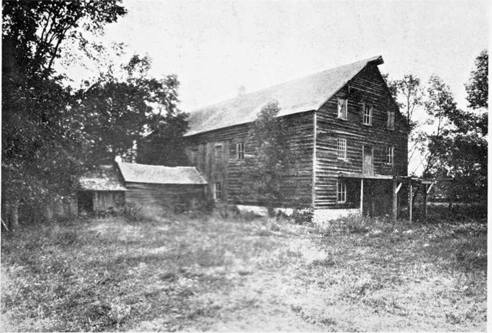
The Asselstine Woollen Mill, the only mill left whose water wheel turns its machinery today as it has done since 1810.
