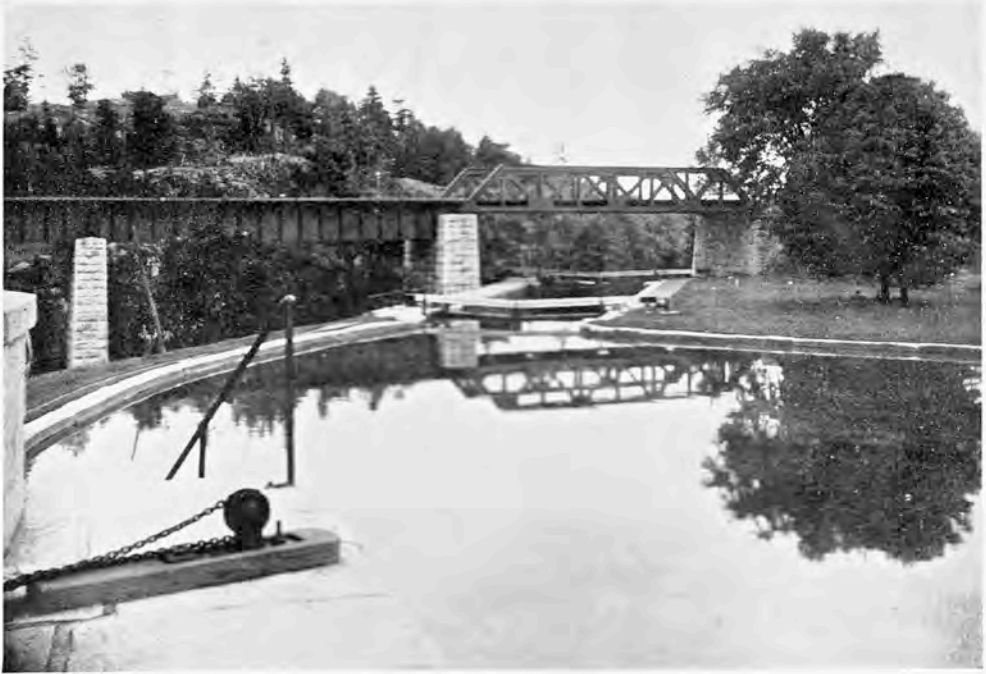
"The Basin", Kingston Mills, showing, at right, the maulting boxes under which the old mill-stone lies, and the second lock.
